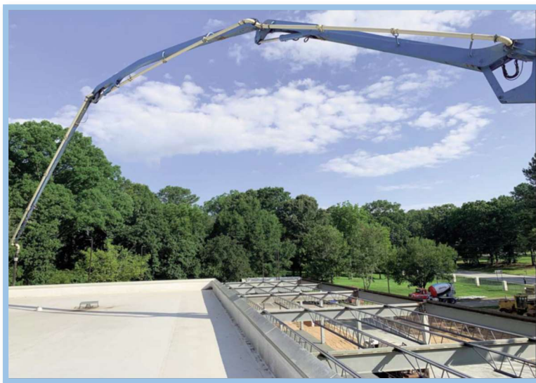
Figure F Construction of new USAPEEC’s Headquarters
